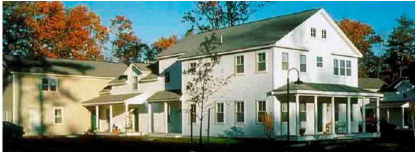
Handicapped accessible multi-family units can be designed to resemble traditional farm structures.
