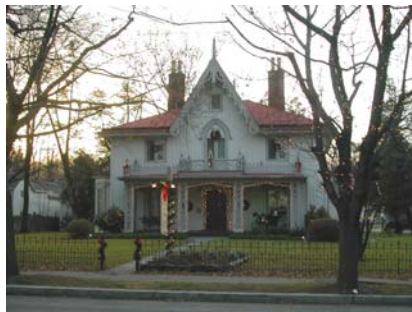
Historic Delamater House
