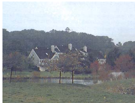
A stormwater management pond is hidden behind dwellings and landscaped to appear as if it is part of the natural setting.
